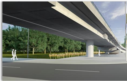
Elevated Guideway - $123M/mile
